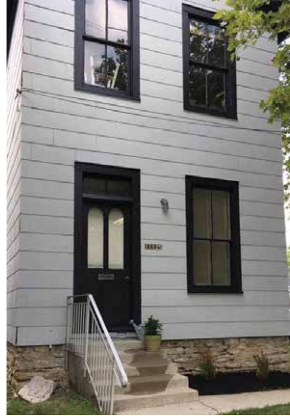
Kimble Mandolins in Downtown Sharonville went through an exterior renovation as a result of being awarded with an improvement grant.
