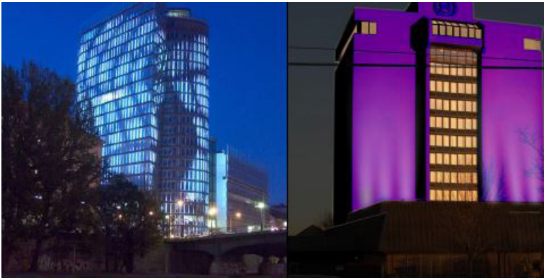
Examples of Building Façade Lighting
